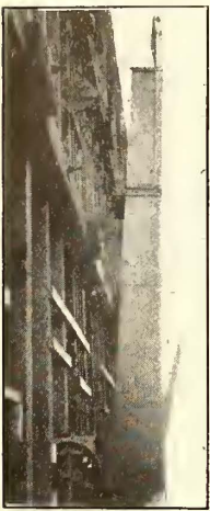
METAL CHUTE FOR DISCHARGING COAL ONTO BARGES
