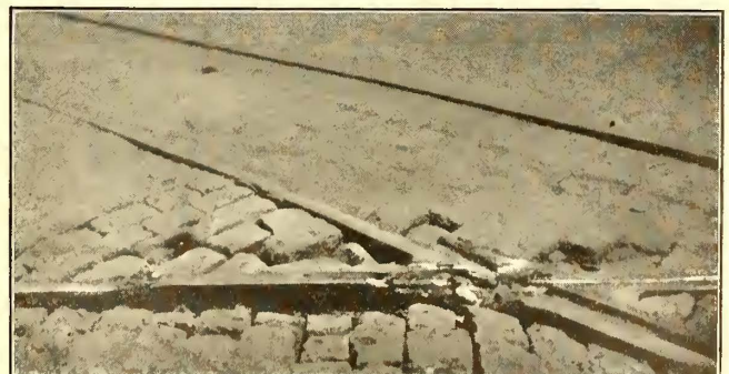
FIG. 4—SAME FROG AFTER WING RAIL HAD BEEN REPLACED WITH NEW RAIL SECTION
