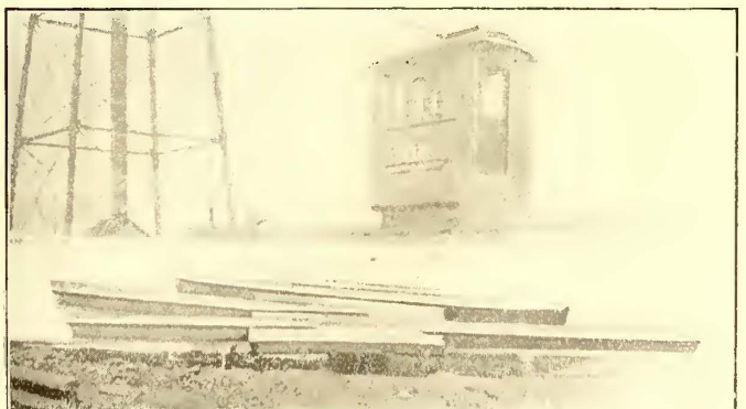
FIGS. 7 AND 8—STANDARD SWITCH-MATE WITH BROKEN THROUGH-RAIL, AND AFTER BEING REPAIRED
