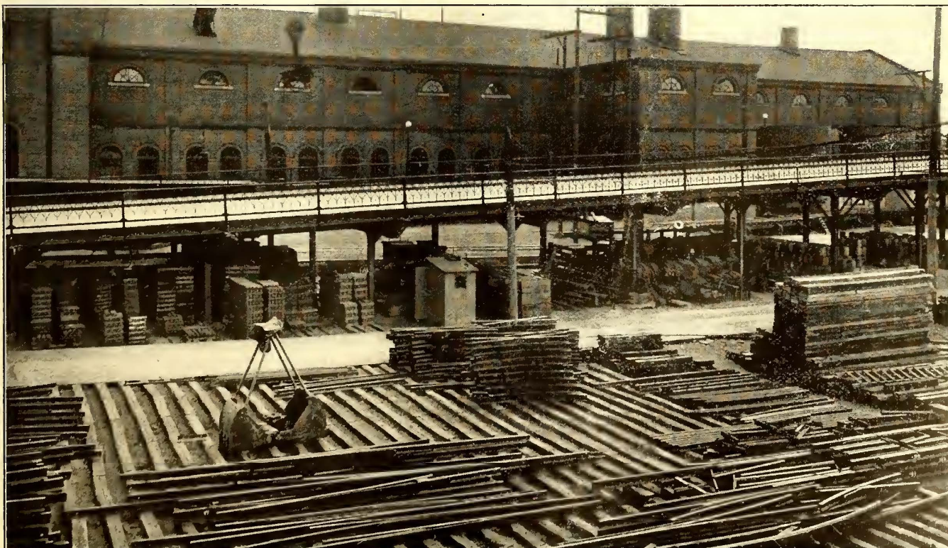
DENVER STORAGE YARD—FIG. 7—SHOWING MATERIAL PILED UNDER VIADUCT
