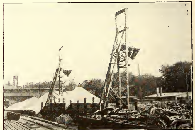
BALLAST-DISTRIBUTING RIG AT PITTSBURGH RAILWAYS' STORAGE YARD
