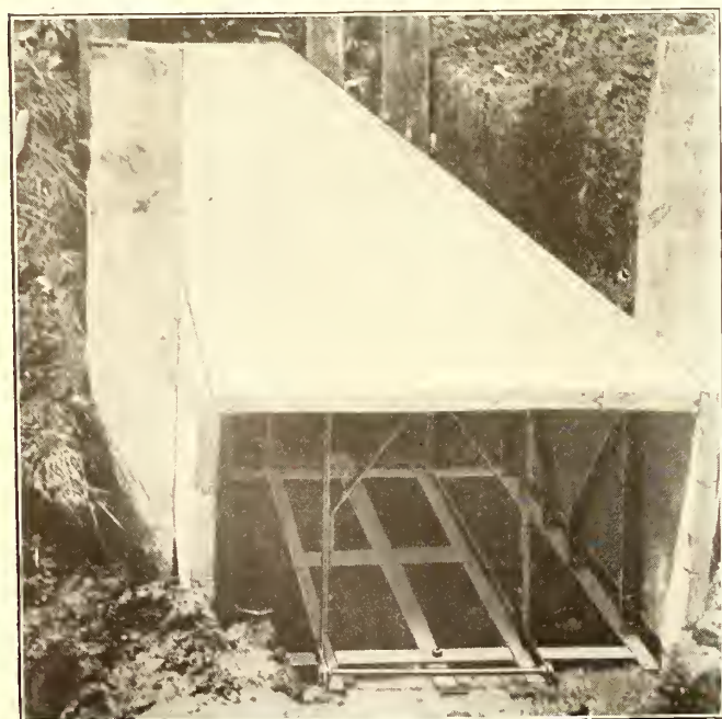
COLLAPSIBLE FORM IN PLACE WITH CASING BOARDS READY FOR CONCRETE
