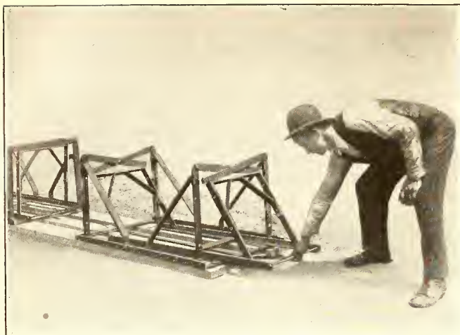
PULLING BOTTOM BAR COLLAPSES FORM FROM THE TOP
