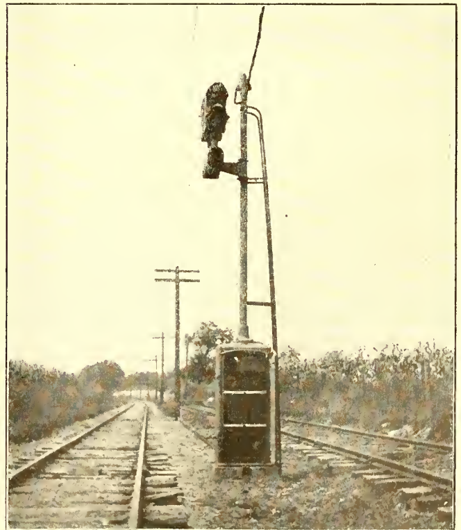
T. H., I. & E. SIGNALS—DOUBLE SIGNAL AND RELAY HOUSING. REAR VIEW
