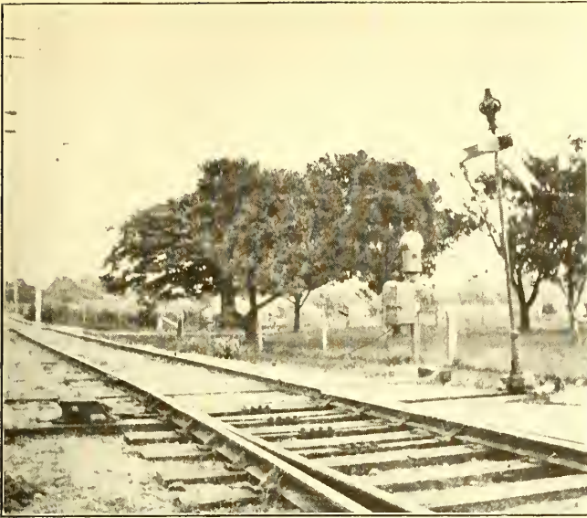
T. H., I. & E. SIGNALS—SWITCH INDICATOR SIGNAL WITH HOUSING FOR TIME-ELEMENT RELAY
