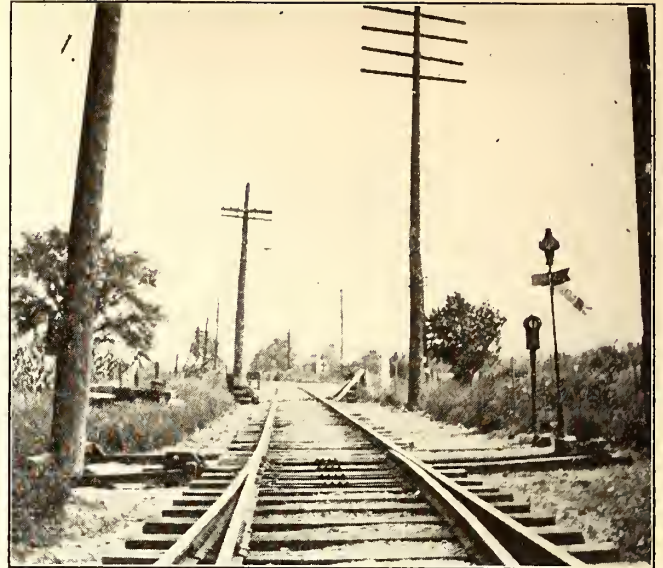
T. H., I. & E. SIGNALS—SWITCH INDICATOR AND SWITCH BOX
