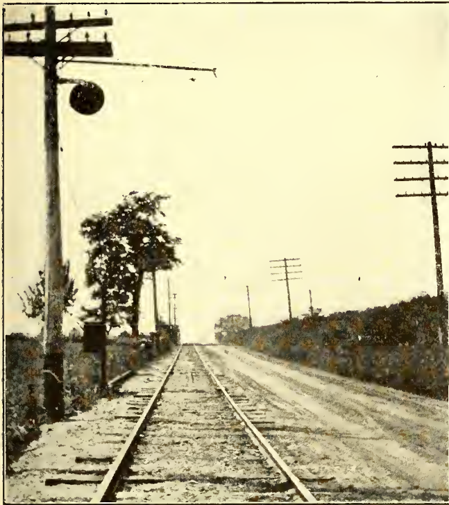
T. H., I. & E. SIGNALS—BLOCK INDICATOR AT END OF PRELIMINARY—THE PURPOSE OF THIS INDICATOR IS DESCRIBED ON PAGE 892
