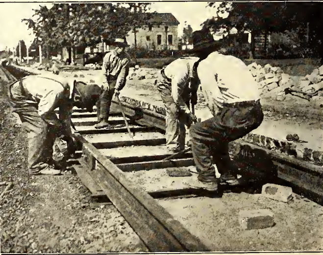
STARTING THE LAST WEDGE BEHIND THE TIE CLIP
