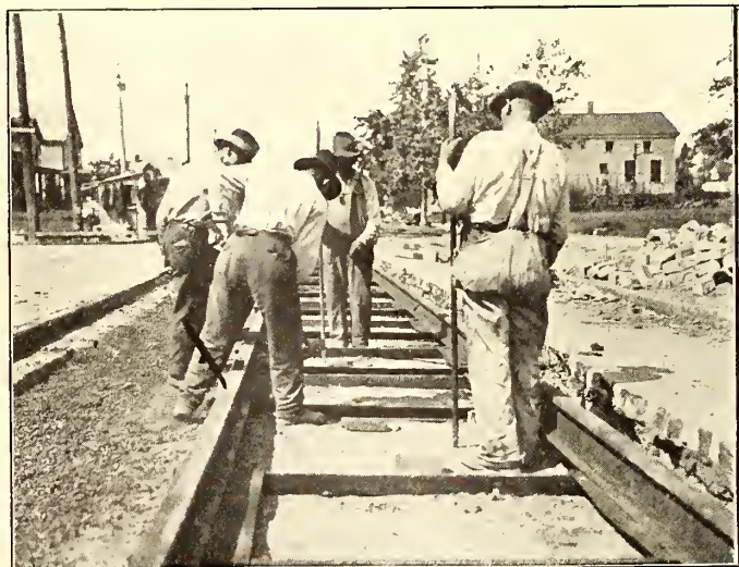
FORCING THE CLIPS AGAINST THE RAIL WITH A SMALL WEDGE
