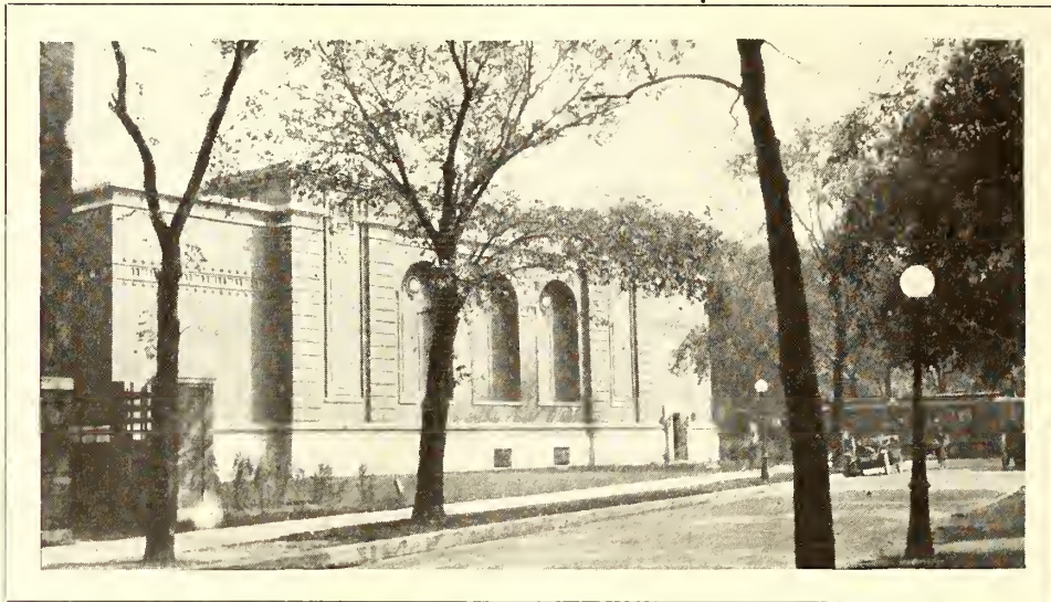
CHICAGO SUBSTATION—PLEASING ARCHITECTURE AND ATTRACTIVE LAWN AID IN OVERCOMING STIGMA OF SUBSTATION
