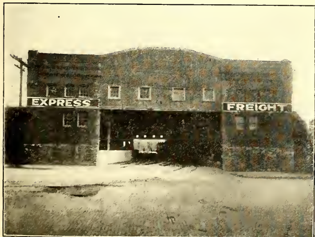
KANSAS CITY FREIGHT TERMINAL—NORTH END OF UNION STATION
