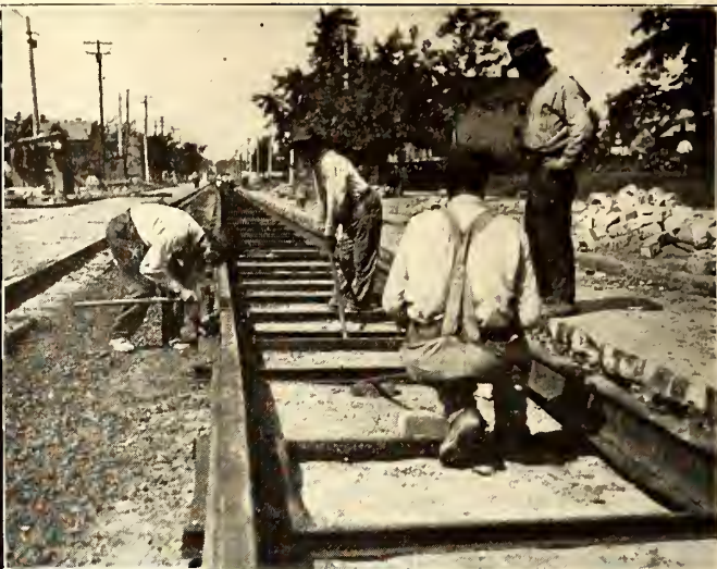
PLACING THE OPPOSITE CLIPS IN THE STEEL TIES
