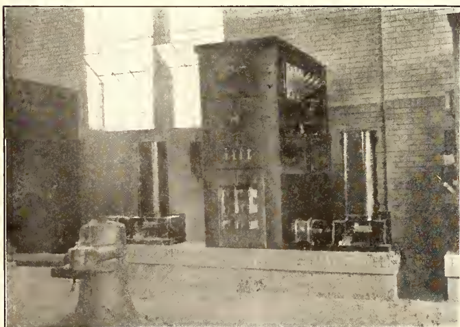
IOWA AUTOMATIC HYDROELECTRIC PLANT—EXCITER CABINET AND MOTOR-OPERATED DRUM CONTROLLER WITH SIDE CASING OPEN TO SHOW CONSTRUCTION
