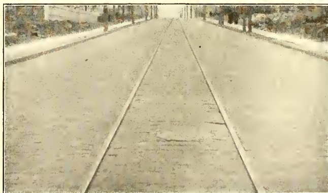
FIG. 2—STANDARD HIGH T-RAIL A.E.R.A. SECTION AS LAID IN FORT LEE, N. J.—SECOND CHOICE
