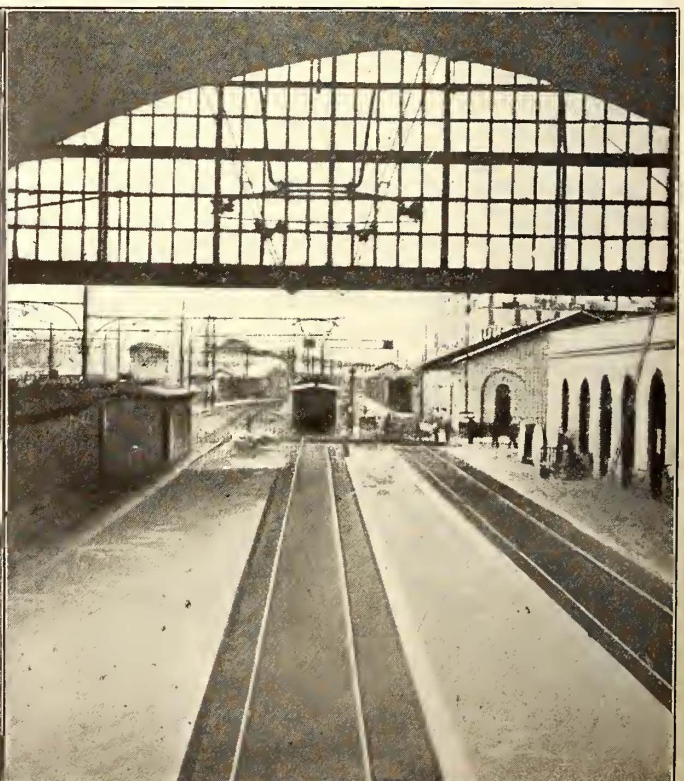
VIEWS OF CONTACT LINE FROM TUNNEL AND CONTACT LINE SUSPENSION AT SAVONA STATION, SAVONA-CEVA RAILWAY
