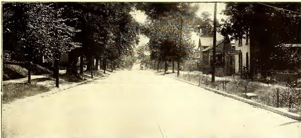
Second Street, looking east from Elm Street, Fort Madison, Iowa. Brick pavement filled with Barrett's Paving Pitch
