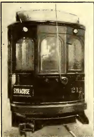
FRONT OF EMPIRE STATE REMODELED CAR, SHOWING CLASSIFICATION BULL'S EYES, AND LONG TRAIL CAR TRANSFORMED INTO INTERURBAN MOTOR CAR
