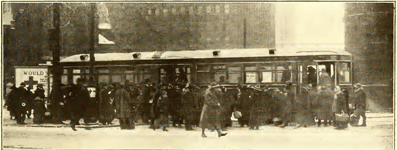
A HEAVY LOADING AND UNLOADING POINT IN BUFFALO, N. Y. WITH THIS TYPE OF CAR THE BOARDING AND ALIGHTING PASSENGERS ARE SEGREGATED
