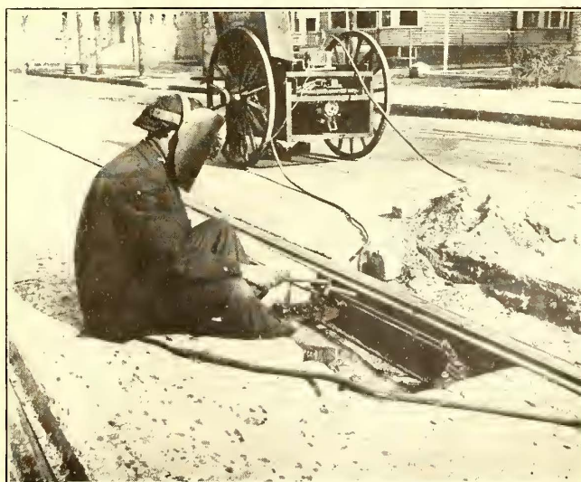
FIG. 6—WELDING RAIL JOINTS WITH THE ELECTRIC ARC
