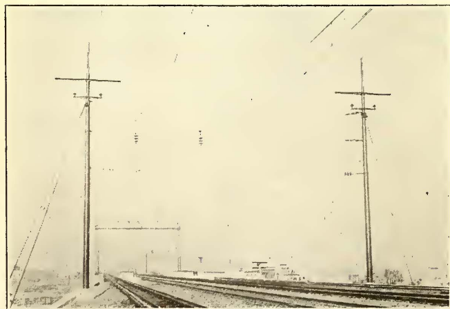
STANDARD SPAN CONSTRUCTION, NEW YORK CONNECTING RAILROAD
