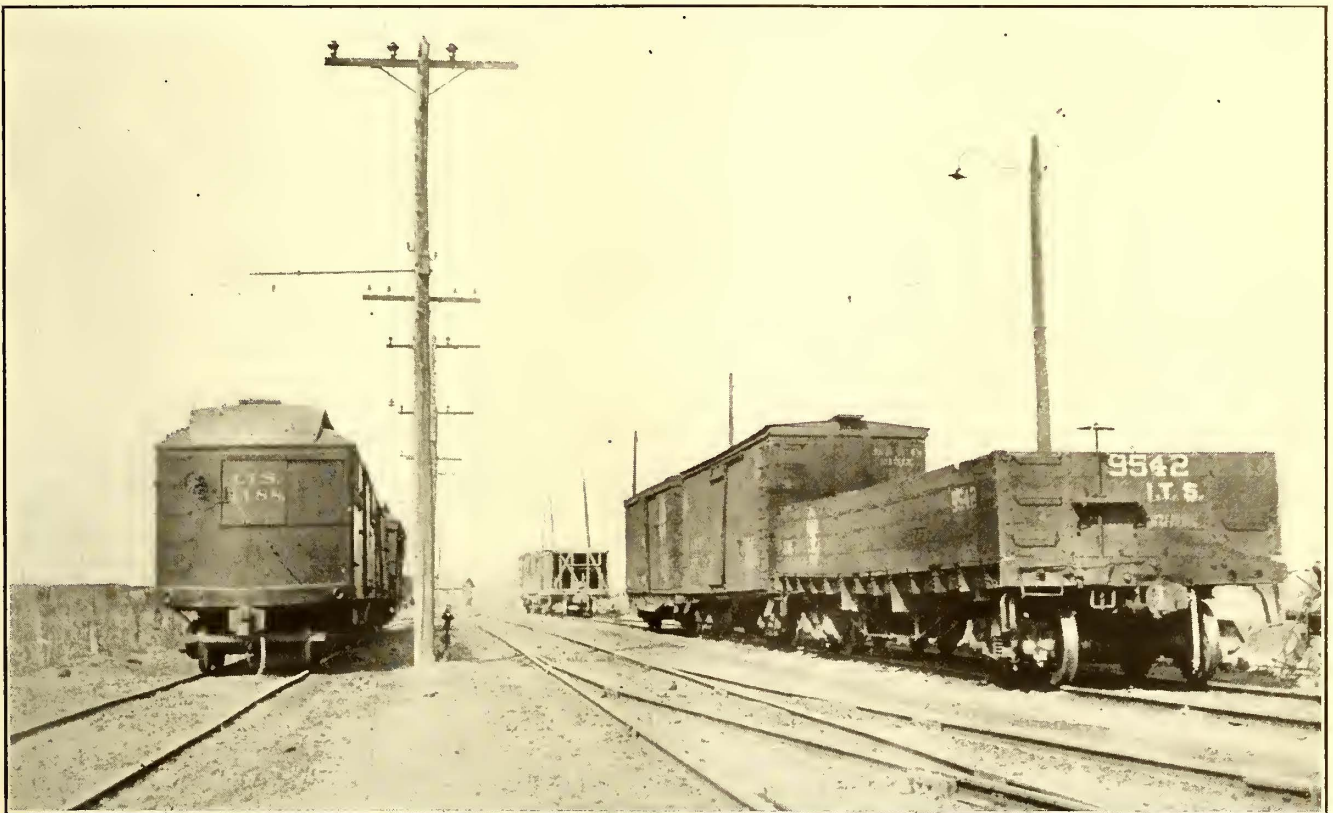
ILLINOIS TRACTION SYSTEM—FREIGHT ROLLING STOCK ALONG A TYPICAL BELT LINE
