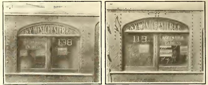
CLEAR WINDOWS WHERE GUTTERS ARE APPLIED, AND STREAKED WINDOWS RESULTING FROM ABSENCE OF GUTTERS
