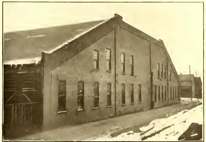
END AND PART OF ENTRANCE TO INSPECTION SHOP
