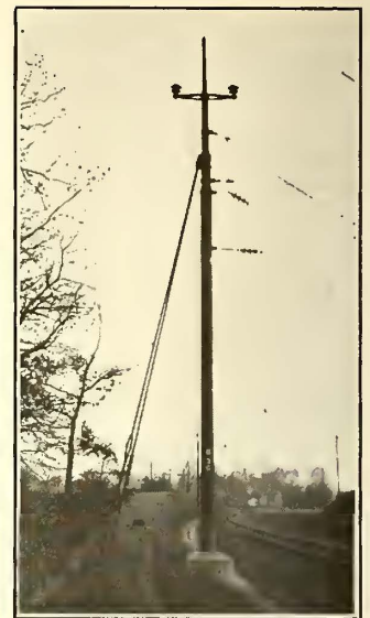
AT LEFT, STUB TOWER FOOTINGS PROTECTED BY CONCRETE CASTINGS (Note how protection has been broken; this is the chief difficulty with this type of footing), AT RIGHT, HEAVY TUBULAR POLE WITH ROD GUYS, PENNSYLVANIA RAILROAD, PHILADELPHIA ELECTRIFICATION
