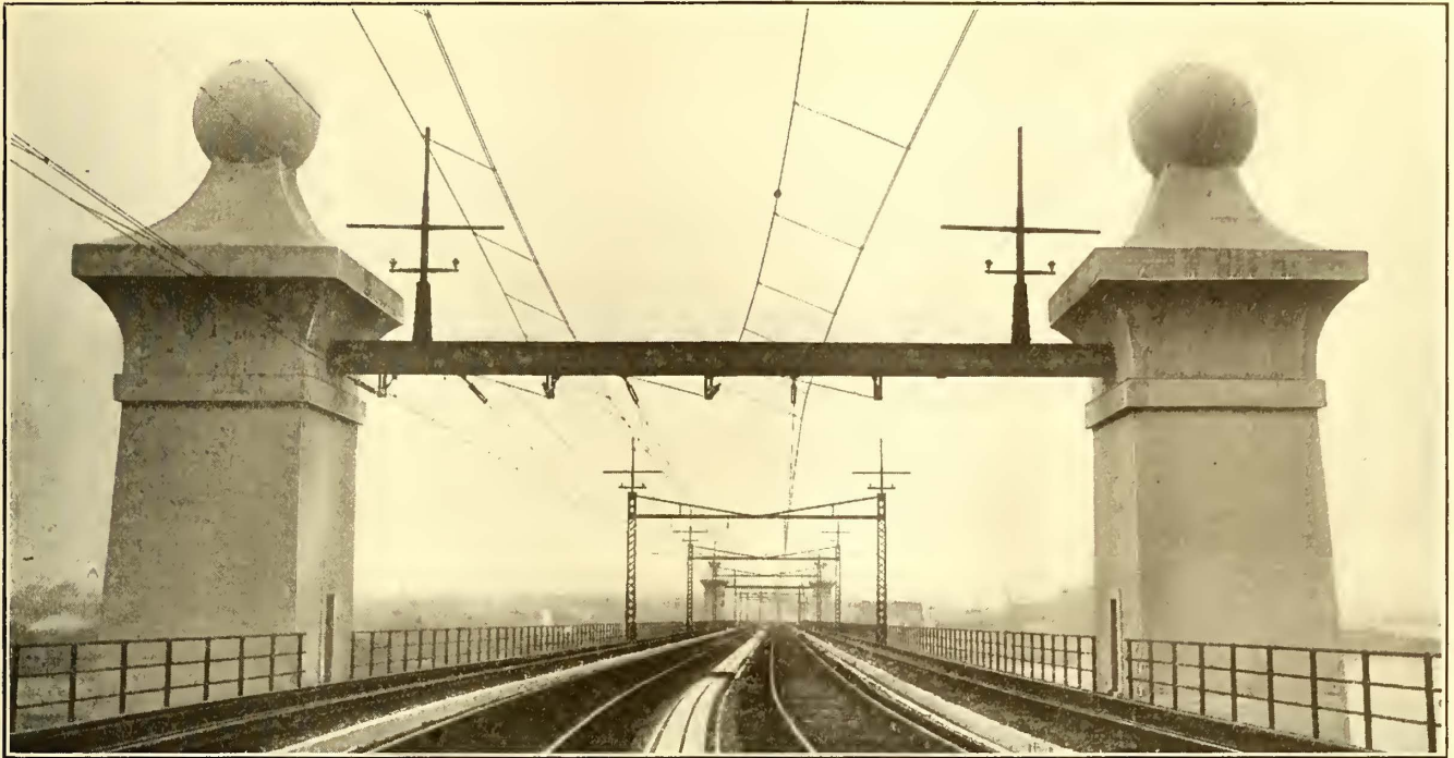
PORTAL AT SOUTHERN END OF LITTLE HELL GATE BRIDGE SHOWING CROSS BEAM AND SAFETY ANCHOR FOR TROLLEYS
