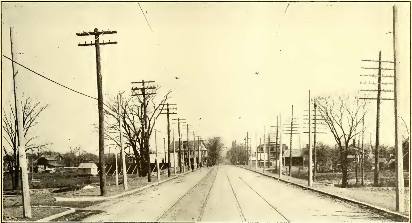
SPAN WIRE CONSTRUCTION WITH CONCRETE POLES, NEW YORK STATE RAILWAYS, ROCHESTER LINES. THIS COMPANY HAS MANY SUCH POLES IN USE
