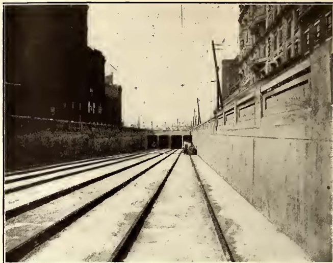
APPROACH TO LOWER LEVEL, SHOWING TRACK UNDER CONSTRUCTION AND CONCRETED IN
