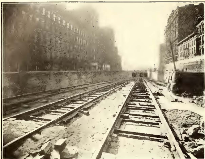
APPROACH TO LOWER LEVEL, SHOWING TRACK UNDER CONSTRUCTION AND CONCRETED IN
