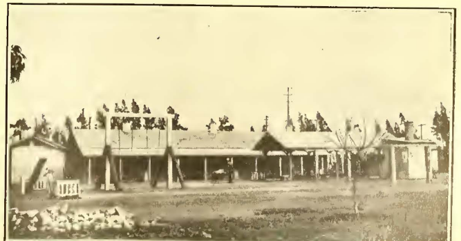
GENERAL VIEW OF SECTION HOUSES AT CULVER CITY CAMP—PACIFIC ELECTRIC RAILWAY
