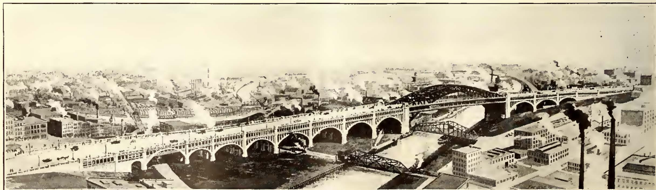
BIRD'S-EYE VIEW OF THE DETROIT-SUPERIOR BRIDGE
