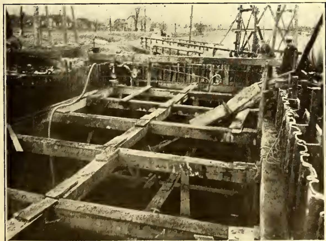
SHEET PILING COFFER-DAM FOR BRIDGE PIER, TONAWANDA CREEK
