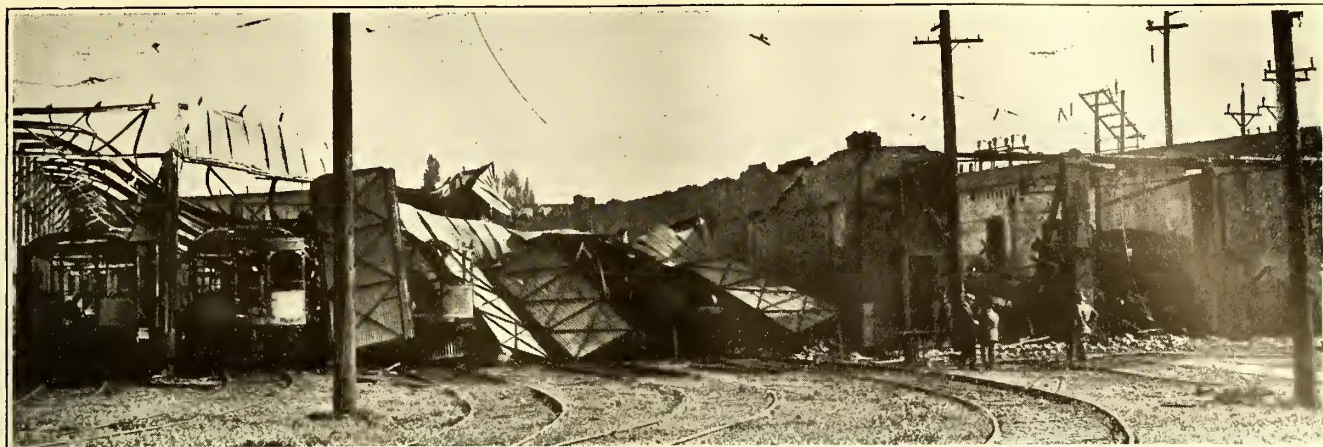
FRONT END OF CARHOUSE AFTER THE FIRE. THE SUBSTATION WHERE THE FIRE STARTED IS LOCATED ON THE EXTREME RIGHT
