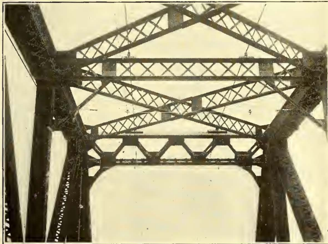
CLOSE-UP VIEW OF OVERHEAD SUSPENSION AND STEADY SPAN ON BRIDGE
