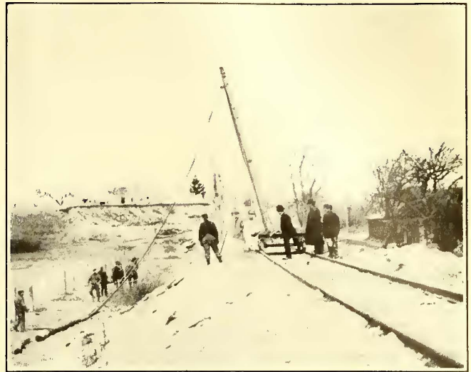
SETTING POLES BY CAR DERRICK—POLE HOOKED ON, HORSES HOISTING
