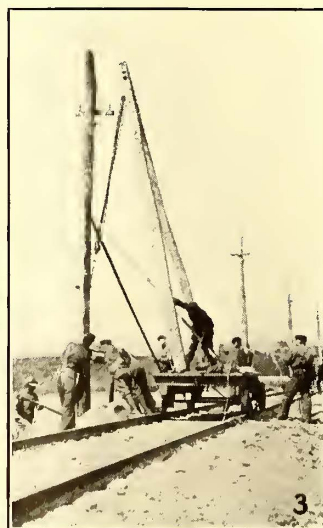
Fig. 1—Pole coming up bank. Fig. 2—Pole nearly up. Fig. 3—Pole in place and nearly lined. Fig. 4—Pole lined, hole being filled SETTING POLES BY CAR DERRICK
