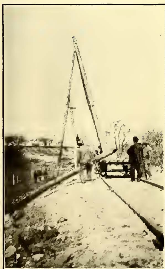
Fig. 1—Pole coming up bank. Fig. 2—Pole nearly up. Fig. 3—Pole in place and nearly lined. Fig. 4—Pole lined, hole being filled SETTING POLES BY CAR DERRICK
