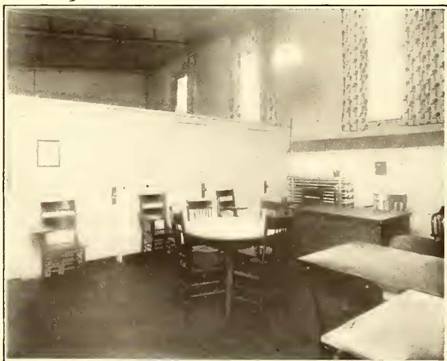
DINING ROOM FOR WOMEN; DORMITORIES AT BACK
