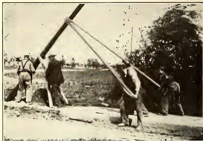
SETTING A STEEL POLE WITH A "JENNEY"
