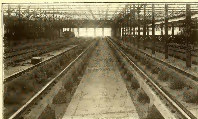
INTERIOR OF TEN-TRACK CARHOUSE AT VICTORIA
