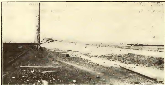
FIG. 5—THE FILL AT THE SOUTH APPROACH OF THE OAK ISLAND VIADUCT
