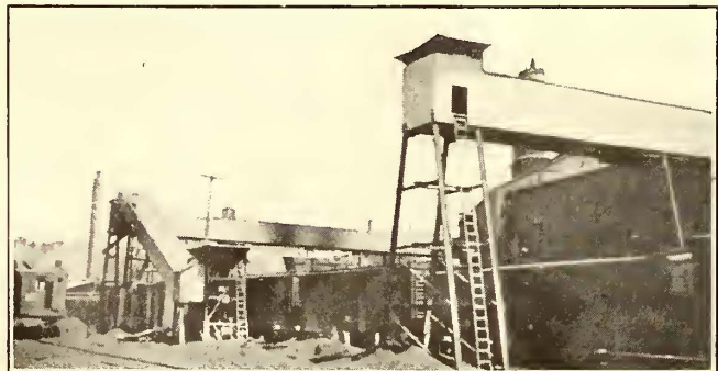
FIG. 2—COAL CONVEYOR EQUIPMENT WHICH WILL HANDLE 80 TONS OF COAL PER HOUR.
