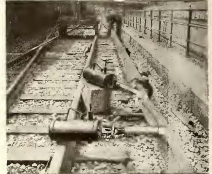
KEROSENE FURNACE BEING USED TO PRE-HEAT A THIRD RAIL BEFORE BONDING
