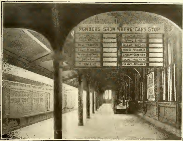
FIG. 1—ELECTRICAL ANNUNCIATOR ON ELEVATED PLATFORM
