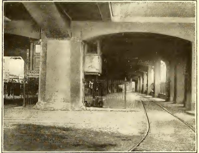
FIG. 2—STATION ENTRANCE SHOWING OPERATING BOOTH AND MOTORMAN'S SIGNAL
