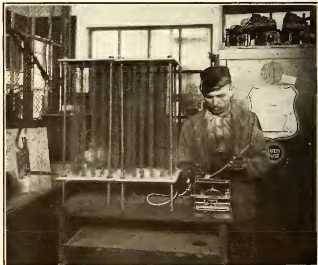
WELDING RHEOSTAT AND BATTERY CHARGING SET
