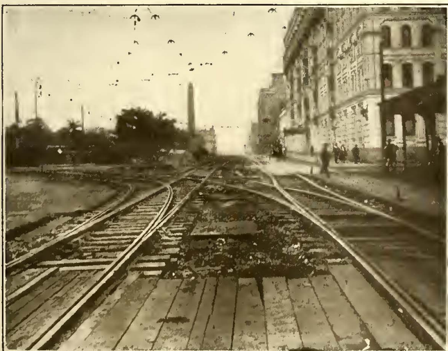
RECONSTRUCTION AND REALIGNMENT OF TRACKS ON ELIZABETH STREET, SYDNEY
