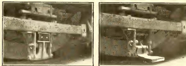
CONTACT SHOE IN RAISED AND RUNNING POSITION
