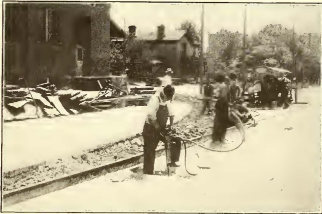
CUTTING OUT CONCRETE AT SALT LAKE CITY, PREPARATORY TO INSTALLING SPUR
