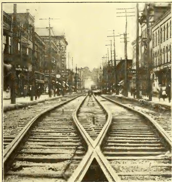
TRACK CONSTRUCTION AT SHARON, PA., BEFORE AND AFTER "PAVING IN"
