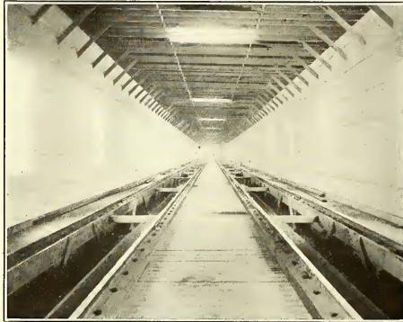
INTERIOR OF INSPECTION SHED AT WHITLOCK AVE.
