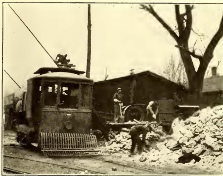
OLD CONCRETE SALVAGED BY PORTABLE STONE CRUSHER AT OMAHA
