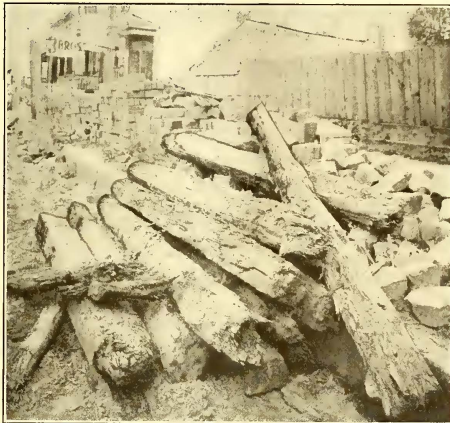
FIG. 6.—TREATMENT WOULD HAVE MADE THESE CEDAR TIES LAST LONGER
