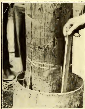
REINFORCING WOOD POLES WITH CONCRETE—AT LEFT, TAMPING THE CONCRETE; AT RIGHT, A FINISHED JOB; IN CENTER, THE REINFORCING OUTFIT ON THE WAY
