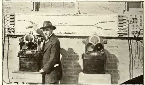
TESTING A PAIR OF SIGNALS BEFORE RETURNING THEM TO SERVICE
