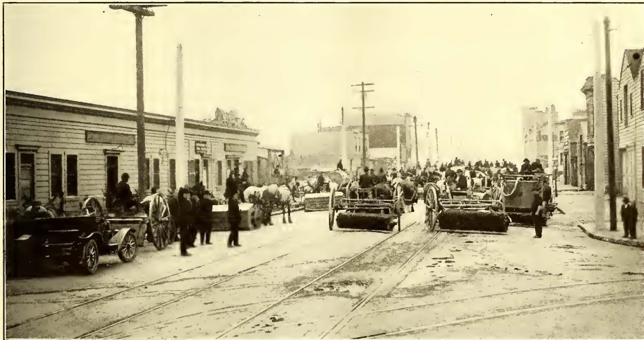
OVERHEAD CONSTRUCTION, SAN FRANCISCO MUNICIPAL RAILWAY, SHOWING CONCRETE POLE CONSTRUCTION
