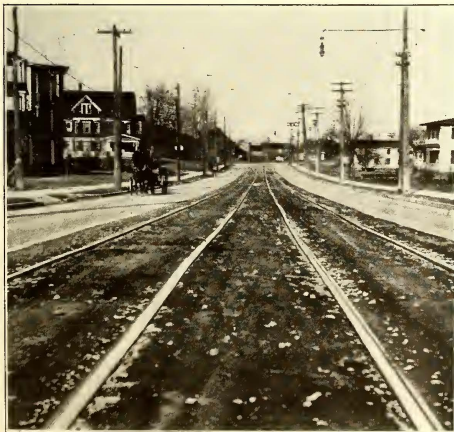
TRACK COVERED BY CASE NO. 3. THIS RAIL IS 9 IN. IN HEIGHT, LAID IN 1894 AND ELECTRICALLY WELDED IN 1909. THE FIRST VIEW WAS TAKEN BEFORE REHABILITATION IN 1918, THE SECOND AFTER REHABILITATION
