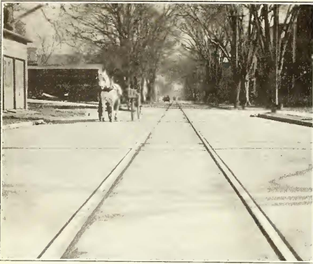
REHABILITATED TRACK COVERED CASE NO. 4
