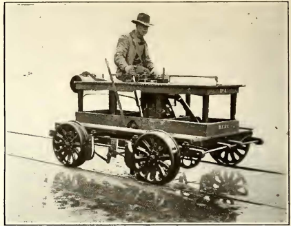
CONTROL SIDE OF CAR SHOWING BRAKE LEVER ON OUTSIDE AND CLUTCH LEVER INSIDE
