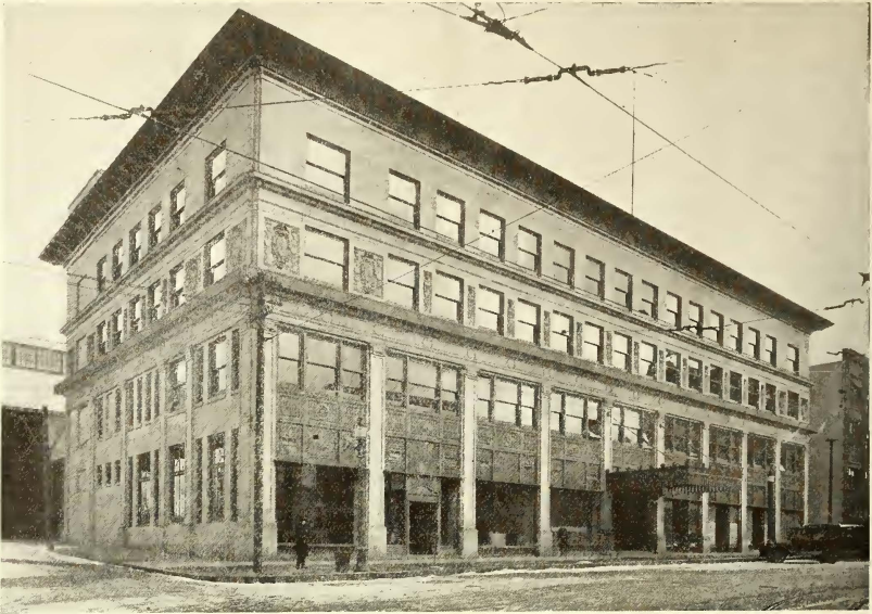
North Main Street Façade of the Office Building, Train Shed in Background
