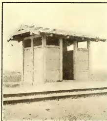
TWO OUTER VIEWS, PASSENGER WAITING SHELTERS OF FRAME CONSTRUCTION TYPE ON PACIFIC ELECTRIC RAILWAY INTERURBAN LINES; CENTER VIEW, UNIT-SLAB CONCRETE WAITING STATION, FORMERLY USED BY THE COMPANY
