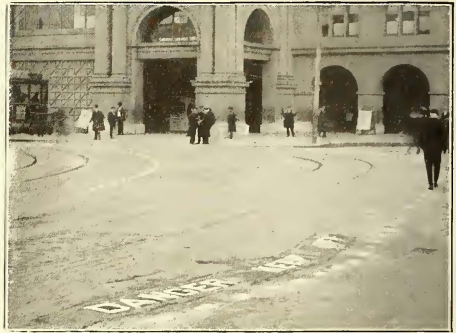
DANGER LINES SHOWN BY WHITE BRICK
