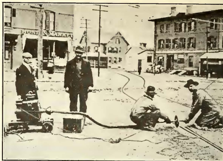
GRINDING A GROOVE IN SPECIAL WORK
