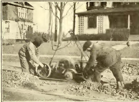
GRINDING A WELDED JOINT WITH A ROTARY GRINDER
