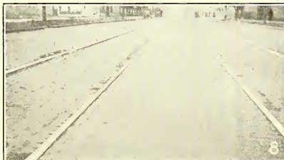
No. 5—Type No. 2A, track laid with mortar cushion in 1911, ties spaced 3 ft.
