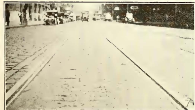
No. 1—Type No. 1, track laid in 1907 with sand cushion
