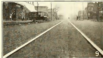
No. 5—Type No. 2A, track laid with mortar cushion in 1911, ties spaced 3 ft.
