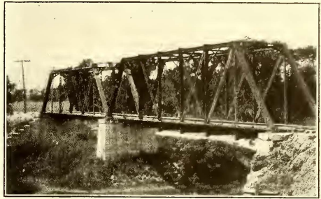
SINGLE TRACK THROUGH TRUSS ELECTRIC RAILWAY BRIDGE
