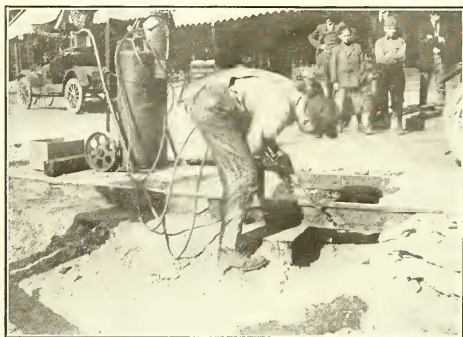
THE NOW FAMILIAR GAS CUTTING TORCH IN OPERATION
