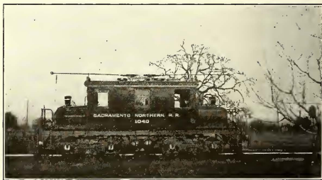
A 50-TON SACRAMENTO NORTHERN FREIGHT LOCOMOTIVE
