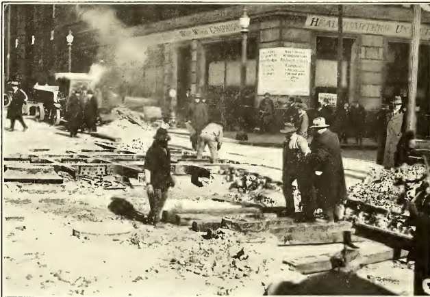
INSTALLING SPECIAL WORK AT BALTIMORE AND CALVERT STREETS
