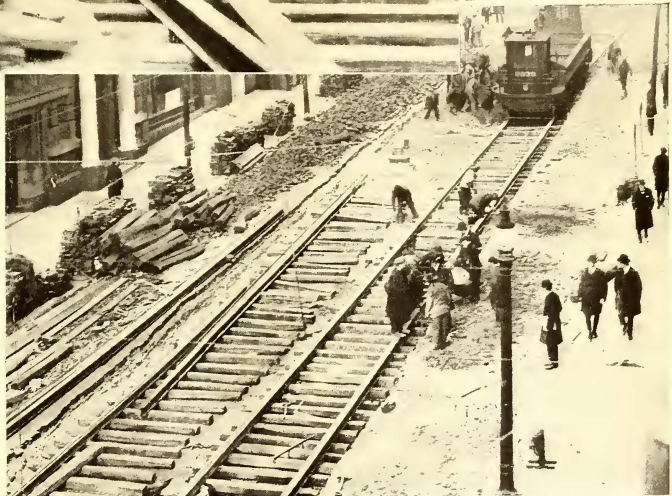
TRACK CONSTRUCTION IN CONNECTION WITH BALTIMORE REROUTING
