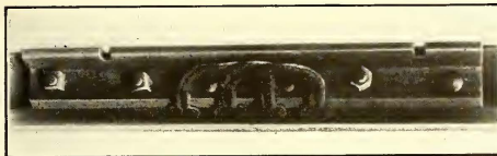
SOLDERED TYPE OF RIBBON BOND FOR HEAD OF RAIL
