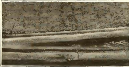
RECONSTRUCTING THE HEEL OF A DAMAGED MATE—AT LEFT, MATE WITH PIECE SHELLED OUT; AT RIGHT, REPAIRED MATE
