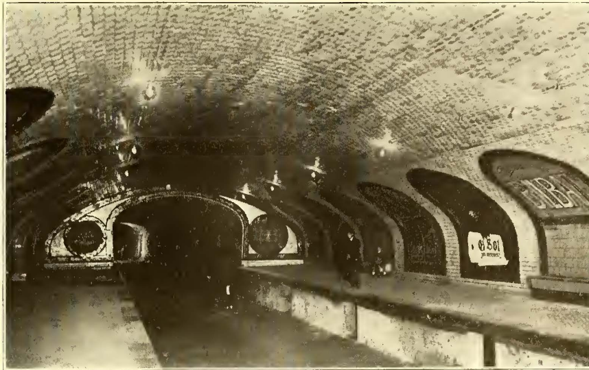
ONE OF THE STATIONS AS COMPLETED
