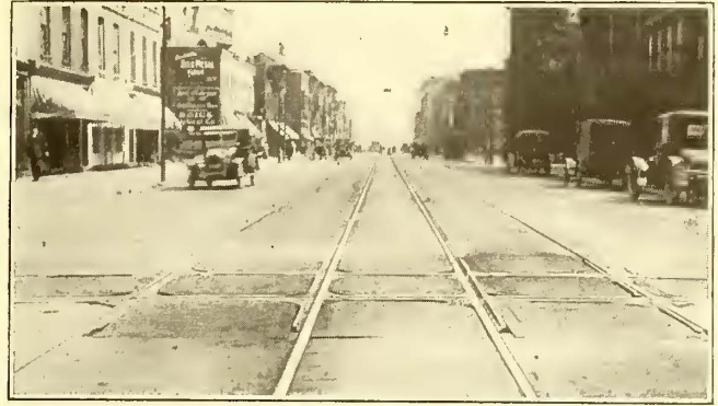
SECTIONAL PAVING CROSSINGS ON THE TOLEDO RAILWAY & LIGHT CO.'S LINE—AT LEFT, INTERSECTION AT CHERRY AND MICHIGAN STREETS; AT RIGHT, INTERSECTION AT CHERRY AND HURON STREETS
