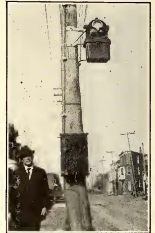
MOUNTING OF SIGNALS AND JUNCTION BOX
