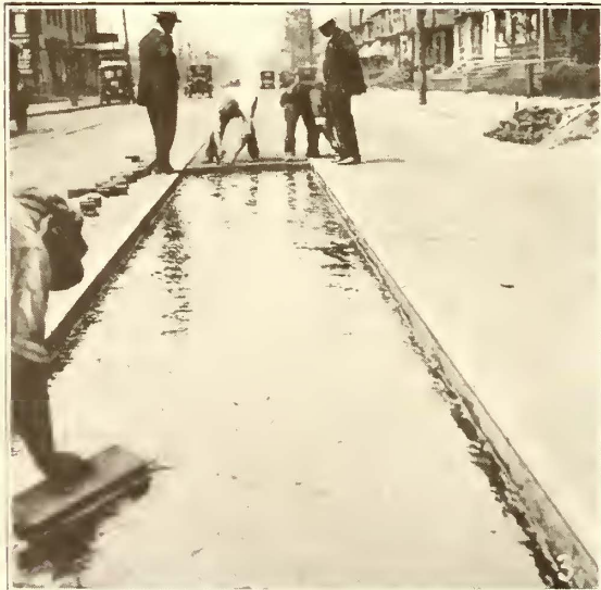
VARIOUS OPERATIONS USED FOR REPAVING BETWEEN TRACKS
