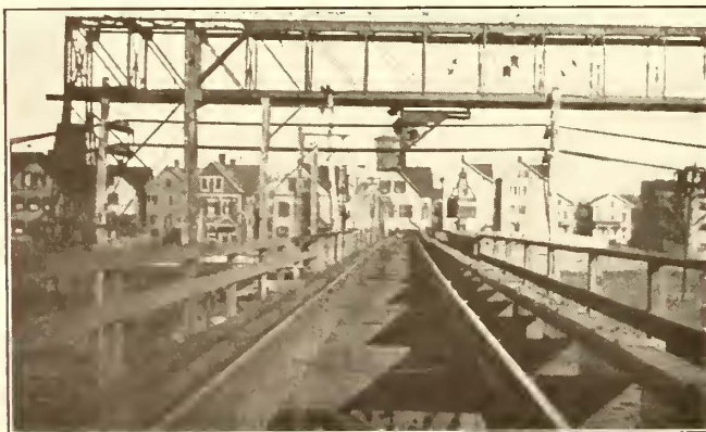
FIG. 6.—TRESTLE AND TRACK EXTENDING THROUGH MAIN STORAGE AREA
