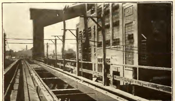
FIG. 7.—LOWERED TRESTLE THROUGH OLD PROPERTY AND THE CONVEYOR WHICH DELIVERS THE COAL
