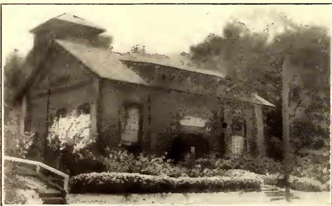
A FRONT YARD FIT FOR A RESIDENCE
