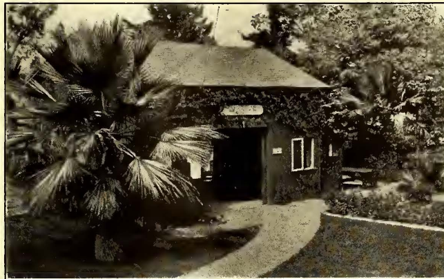
A SUBSTATION SET IN A GARDEN
