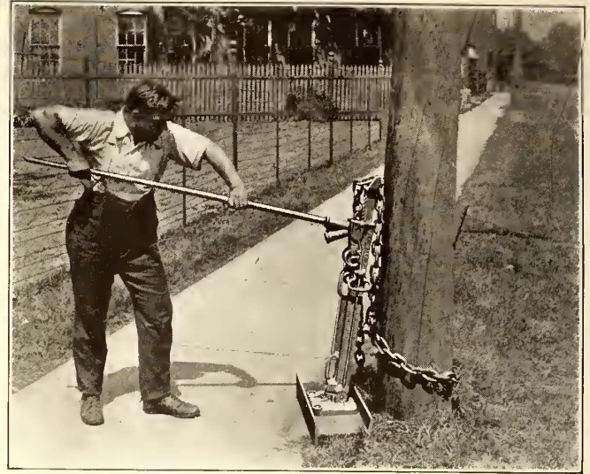
LIFTING A POLE BY MEANS OF A JACK
