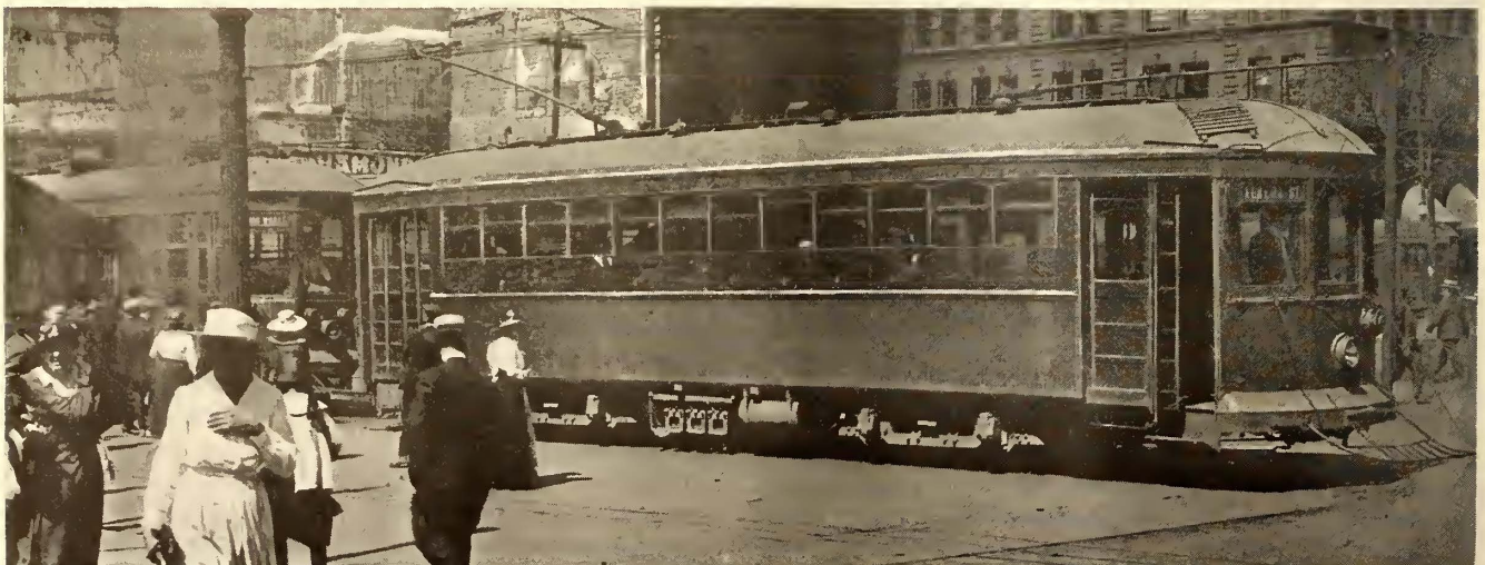
TESTS ON THIS DOUBLE-END CAR HAVE SHOWN THAT THE TIME OF PASSENGER INTERCHANGE WITH IT WAS OVER 50 PER CENT GREATER THAN ON A PETER WITT CAR
